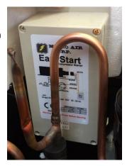
3. Pull back the grey putty around the wires that pass the compressor wires through the plastic air box separator. Pass the braided wires from EasyStart through the hole and form the putty back around the wires and over the hole.
